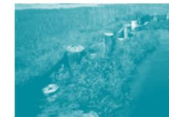
Artificial protection along the margins obstructs the normal relationship between the marshes and the bordering mudflats. This photo shows the tendency of nature to claim her spaces, albeit by colonising extraneous substrates. The step change in height created by the stone-filled sacks does however introduce evident limits to regeneration progress.
